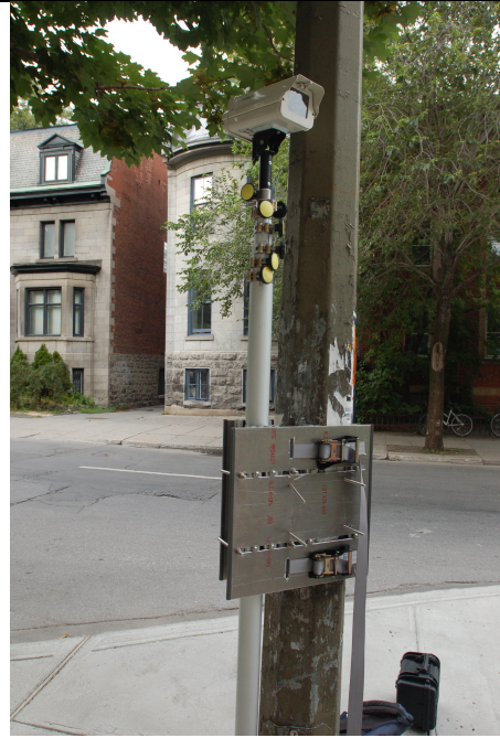
D: Mast Installed On Panel Using Bracket, Ready For Enclosure Installation
